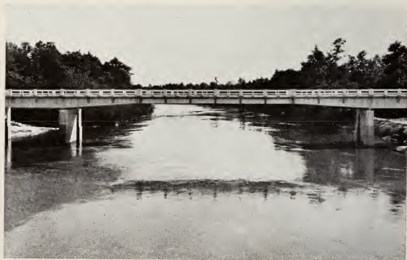
STEEL AND CONCRETE BRIDGE
