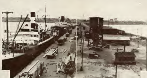
DEEP WATER PORT - GULFPORT
