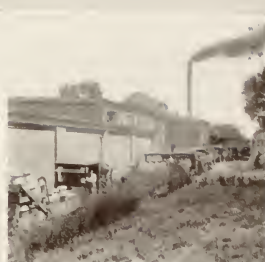
CONDENSED MILK PLANT STARKVILLE —
