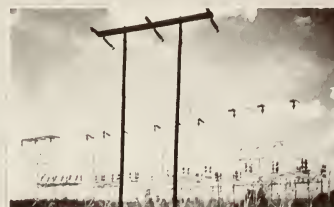
ELECTRIC POWER ~ GREENWOOD
